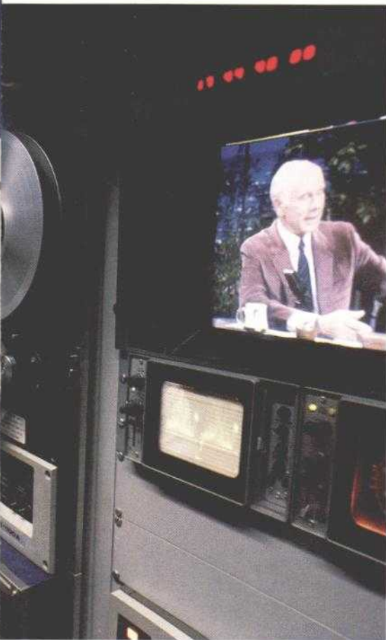
Above, In the Skypath Room at NBC-New York, Central control and monitoring of the Satellite Network Management System (SNMS) for the Comsat General/NBC Distribution System takes place here and in a similar room at NBC-Burbank. The most critical job of the satellite system is the switching function—telling the electronic traffic where to go. Skypath computers are loaded daily with switching information for all of the 181 earth stations in the system. Shown are NBC engineers Stev Asay, left, and Robert J. Butler, Chief Engineer, Satellite Network. Left, Distribution of "The Tonight Show Starring Johnny Carson" to over 200 NBC-affiliated stations starts at this video-feed machine at NBC-Burbank. Broadcast engineer John Griffin operates machine.
