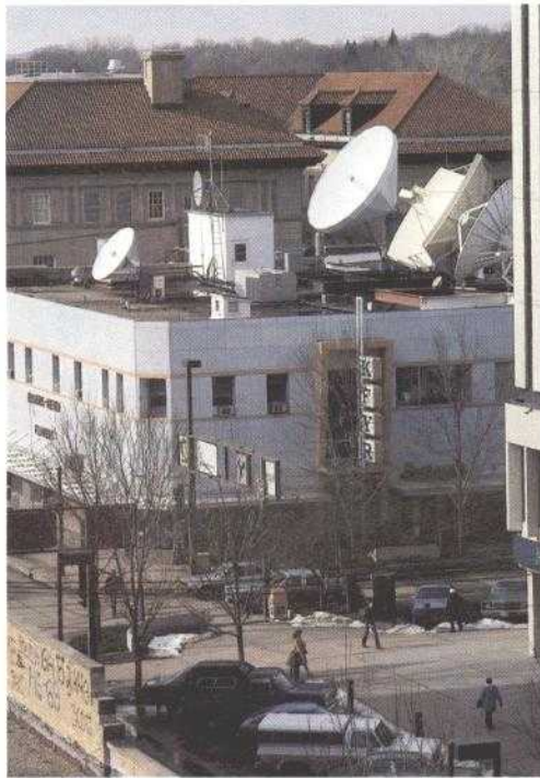
Above, View of NBC affiliate KFYP-TV in Bismarck, North Dakota. Comsat General/NBC Distribution System antennas are two pointed upward to the left on roof of building, the 3-meter backup and 6-meter primary. Below, KFYP-TV station manager is Claire Anine Holmberg, Chief Engineer is Jack Davis.
